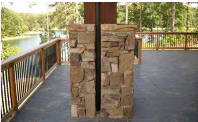
U-channel installed within a mixed column of wood and stone.
