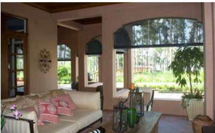
Arched openings with 80% sun block to control UV rays and temperature create a more livable outdoor space.
