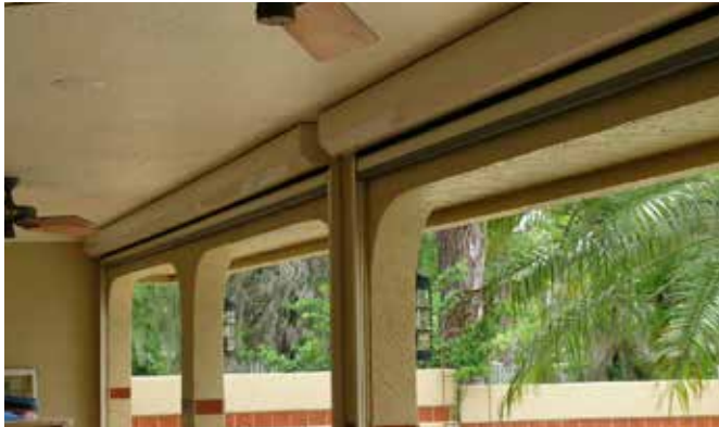
Standard mount motorized screens with housings and standard tracks. Inside above header mount.
