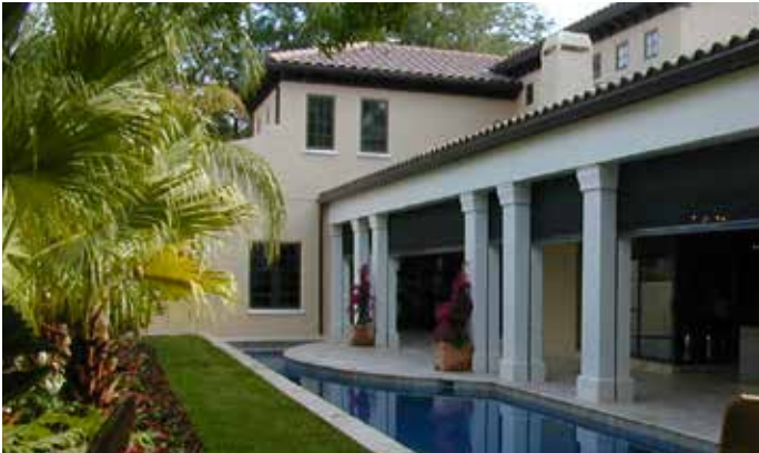
Recessed mount motorized screens built into cavities with recessed U-channel in decorative columns.
